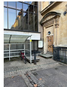
Rear Entrance Crown Road
